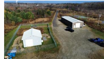
CWD Treatment Facility
