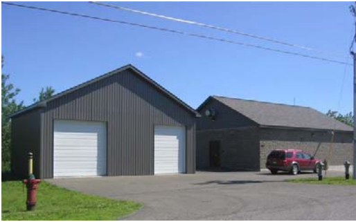
Caribou Water Treatment Plant
