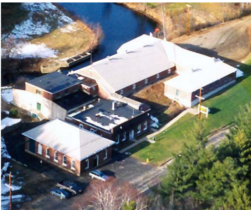
Kennebunk Water Treatment Plant
