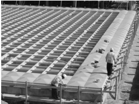
Alignment & Pre-tank assembly works
