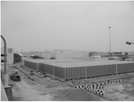
Completed Tanks (17 Feb. 03)
