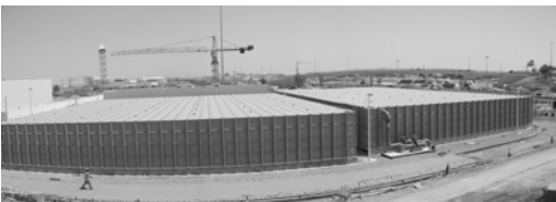
A Panoramic View The Biggest FRP Panel Tanks in the world Capacity : USG 2,500,000
