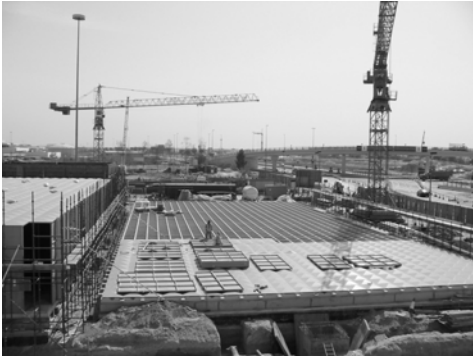
Laying up Bottom Panels on Steel Skid
