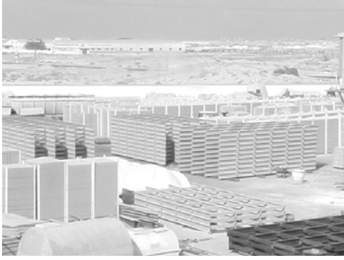
Steel Skid preparation works off-site.
