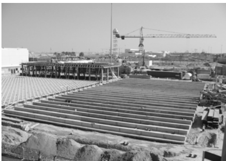
Concrete Foundation Ready (10 Jan. 03)
