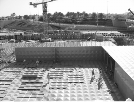
Side & Baffle walls construction
