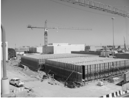
Finishing works (Tie Rods, Air Vents, Ladders, Flanges)
