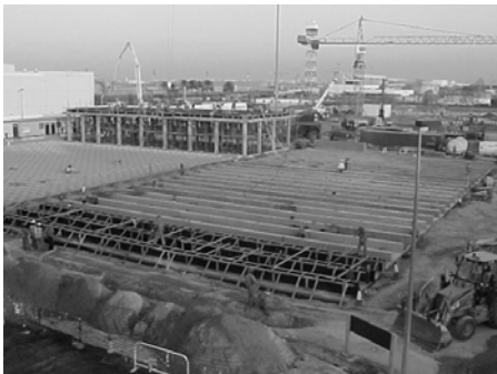
Shuttering for Concrete Foundations
