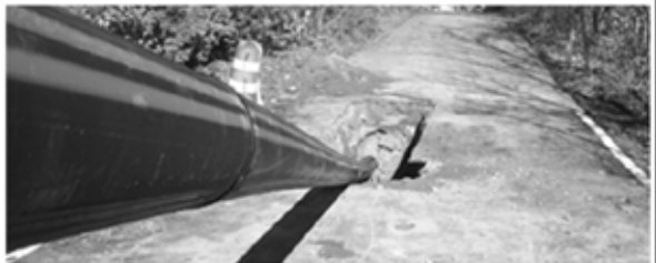
80 Ton Static Burst Machine for bursting long lengths of larger diameter pipe. 6"-16" Solid 2.25" rod
